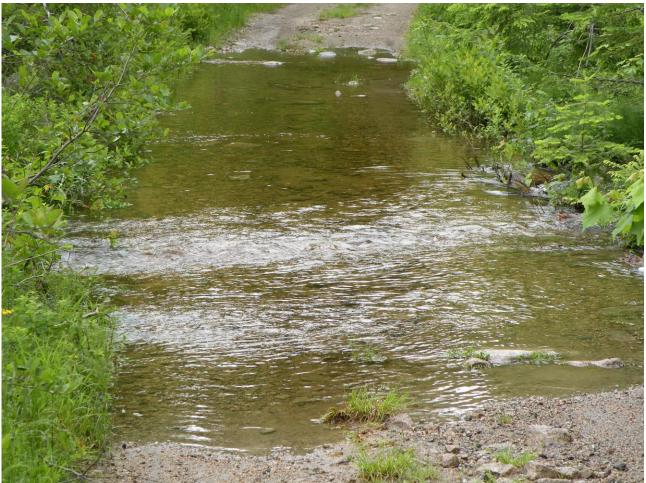
Situations like a blocked culvert shown here cause water to run over roads, picking up sediments that will reduce a lake's transparency.
